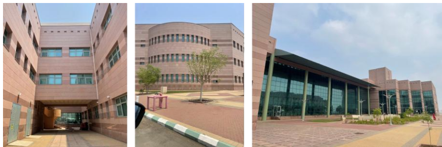
Fig. 4. Multiple views of the CECS building at Jazan University (Photo by the authors, September 2024).
