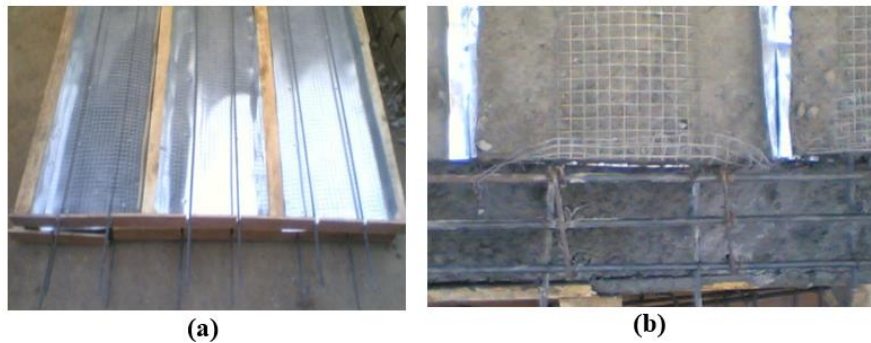
Fig. 20. Anchoring of zinc-coated ferrocement plates on beams: (a) before anchoring and (b) after anchoring.
