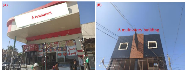
Fig. A-1. Some urban area (Saif Saad district) features, such as a restaurant (A), and a multi-story building (B).
