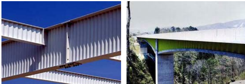
Fig. 1. Some buildings have corrugated beams.
