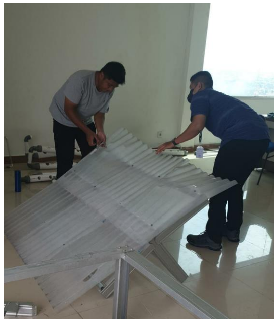
Fig. 2. UV plastic roof installation.
