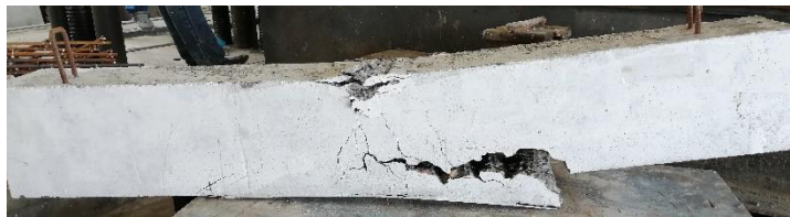
Fig. 8. SB1 Beam delamination.
