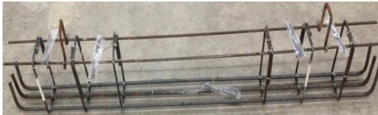
Fig. 3. Steel cage of beam (B1).
