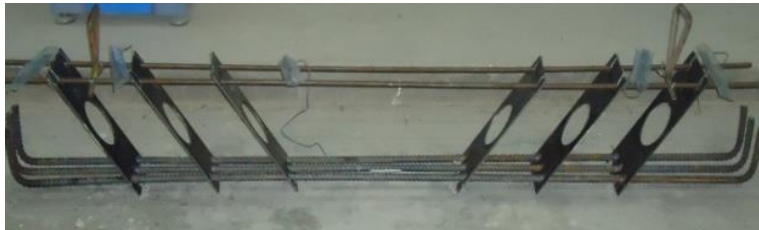
Fig. 4. Steel cage of beam (B2).
