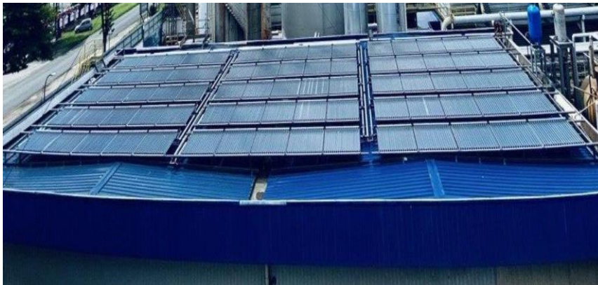
Fig. 1. Evacuated tube collectors (ETC) at SHIP system.
