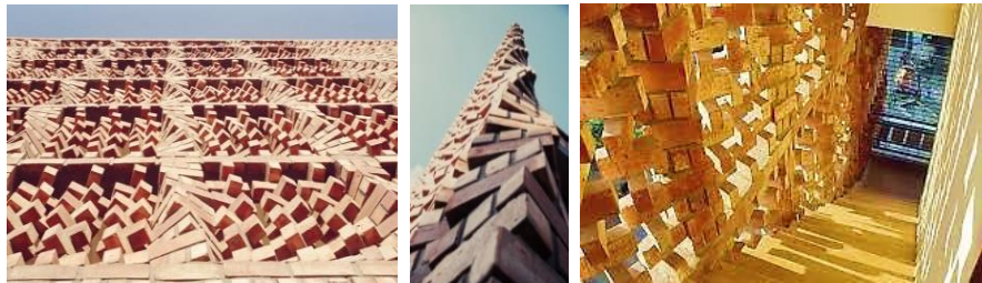
Fig. 8. SAHRDC office building [27].
