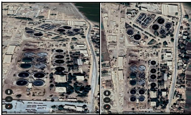
Fig. 2. West of Sohag wastewater treatment plant (source: Google earth).
