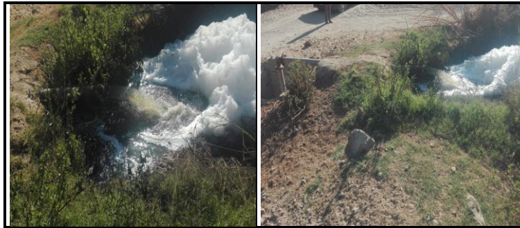
Fig. 5. Outlet of partially treated wastewater at the basin edge (source: site visit).
