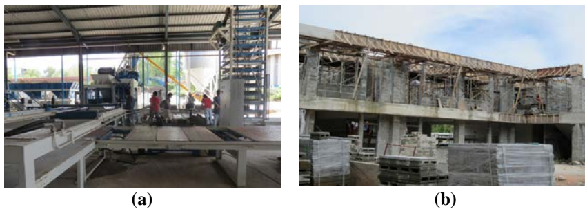
Fig. 5. (a) Production facility of the CMU blocks, (b) Construction site.
