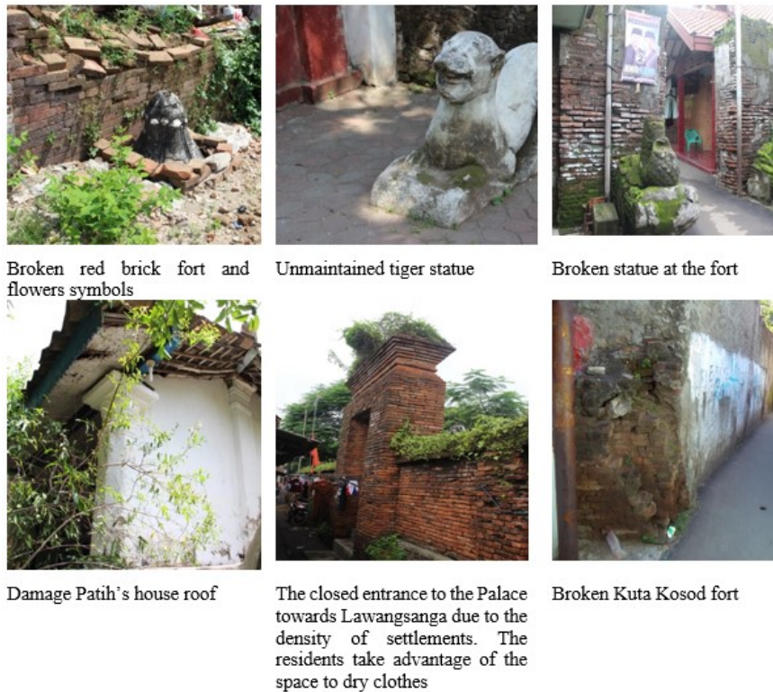
Fig. 5. Damage to palace artifacts in Magersari area.
