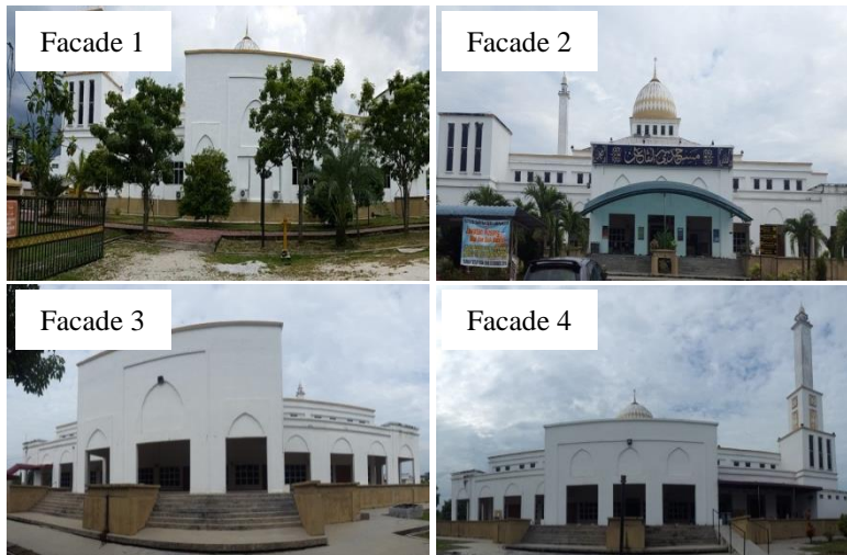
Fig. 5. Views of the mosque’s facades (MQS14).
