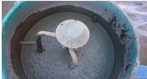
Fig. 4. Self-compacting concrete mixing.
