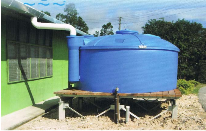
Fig. 2. Rainwater harvesting tank supplied by Weida (M) Bhd.
