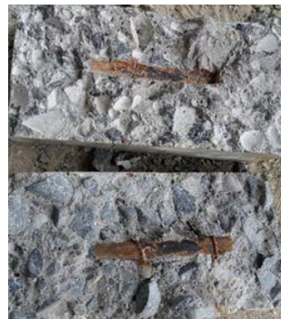
Fig. 4. Removal of embedded steel bar in concrete.
