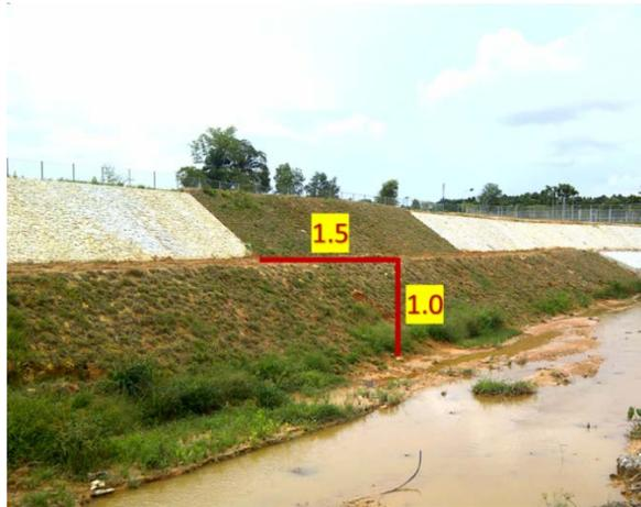
**Fig. 2. Existing slope geometry in Mutiara Rini, Johor.**
