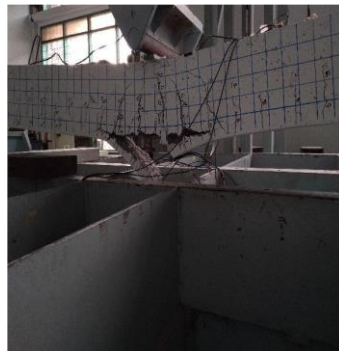
Fig. 5. BU - B1 crack pattern.
