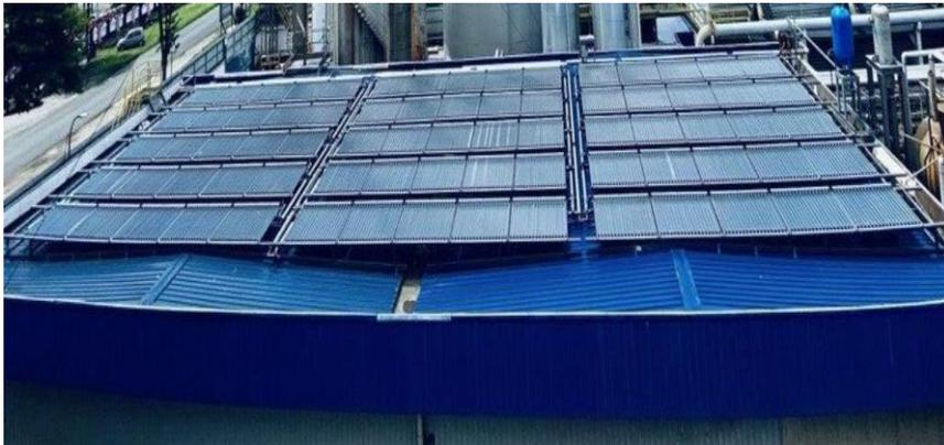
**Fig. 1. Evacuated tube collectors (ETC) at SHIP system.**
