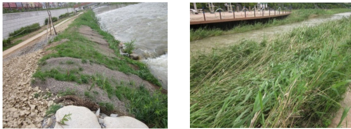
(a) Wash away of Phragmites japonica (b) Collapse of Phragmites japonica Fig. 2. Vegetation Impacts by Flood Flow.
