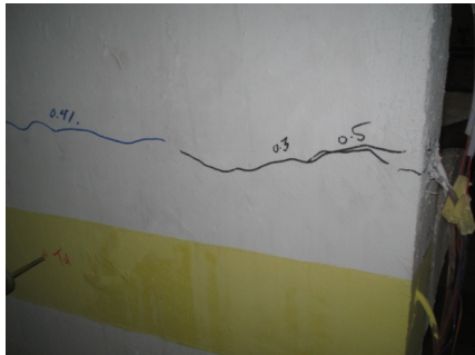
c) Spreading of Cracks across the Wall.
