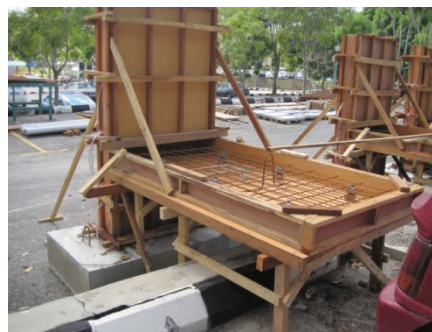
Fig. 4. Formwork Erected on the Foundation Block.
