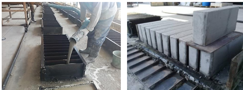
Fig. 1. POFA-foamed concrete blocks production.
