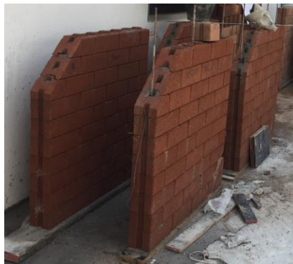
Fig. 4. CCI brick masonry walls.
