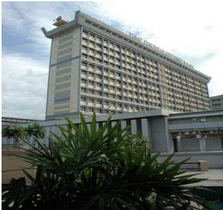
Fig. 1. Overview of the building.
