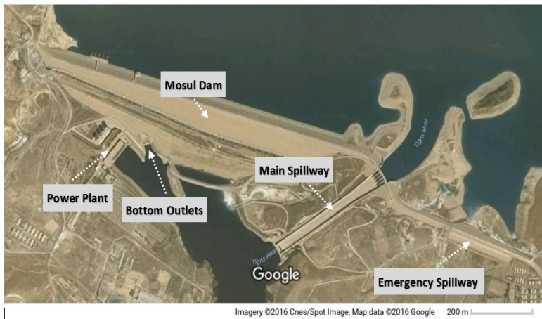
Fig. 3. Mosul dam satellite view.
